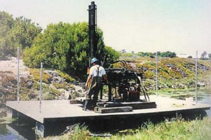
Strataprobe drilling in tidal lagoons, San Diego Bay.
